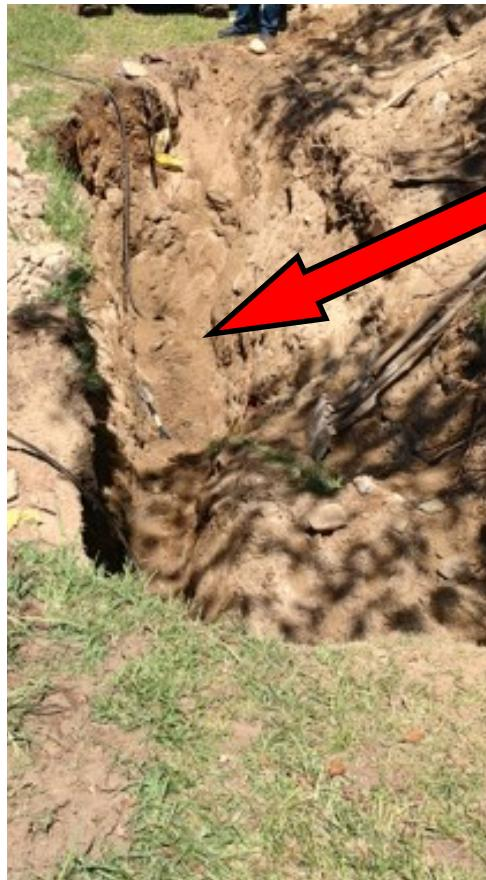
Location of trench cave in and severed natural gas service line. Notice the depth of excavation and lack of shoring or a trench box.
